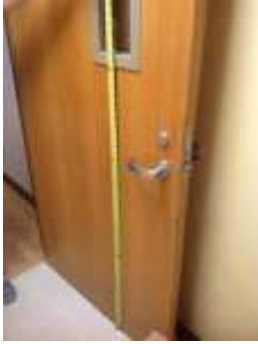
Finding #68, Additional Finding Photos
