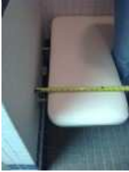
Finding #35, Additional Finding Photos
