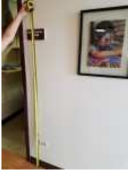
Finding #25, Additional Finding Photos
